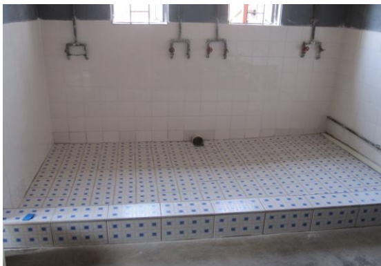
The bathrooms after tiling
